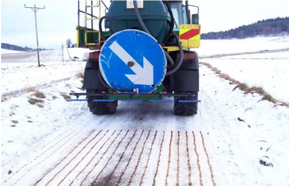
Applying ABP Liquid in longitudinal lines on snow and ice
